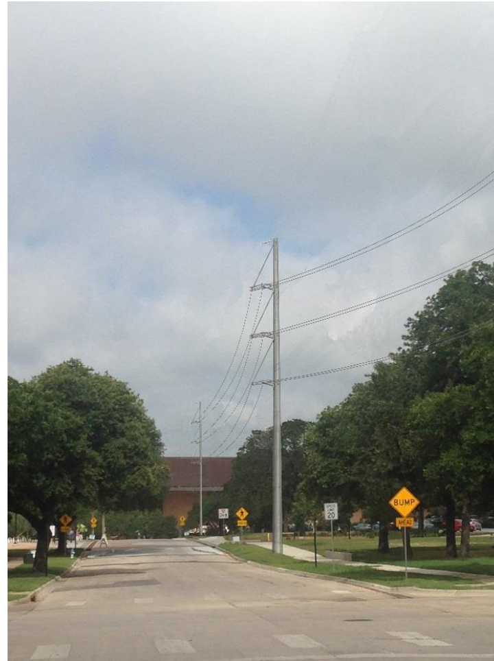
Reduce and Replace Poles
